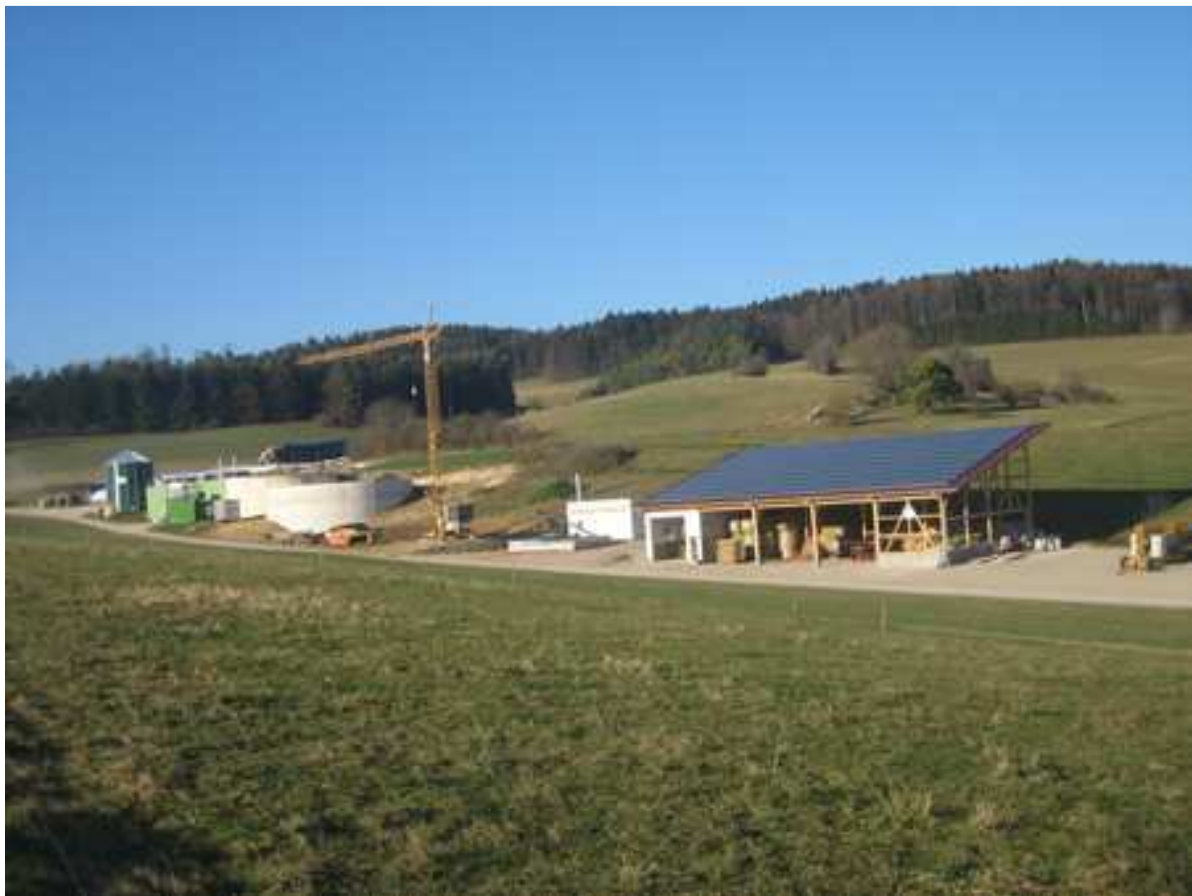
Biogas facility (in the building, woodchip heating system and solar power station)
